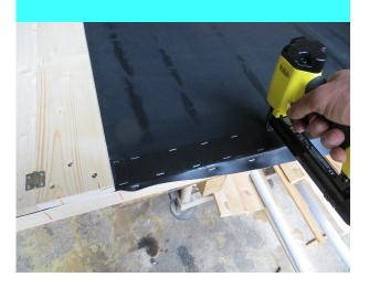
11. Remove the provisional clips from the side of the frame
