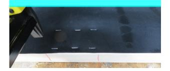
4. Align the hatch and secure the 100 mm board on both ends with three screws.
