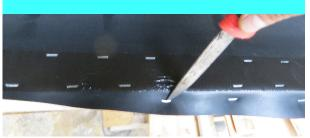
12. Using a sharp knife, remove excess rubber
